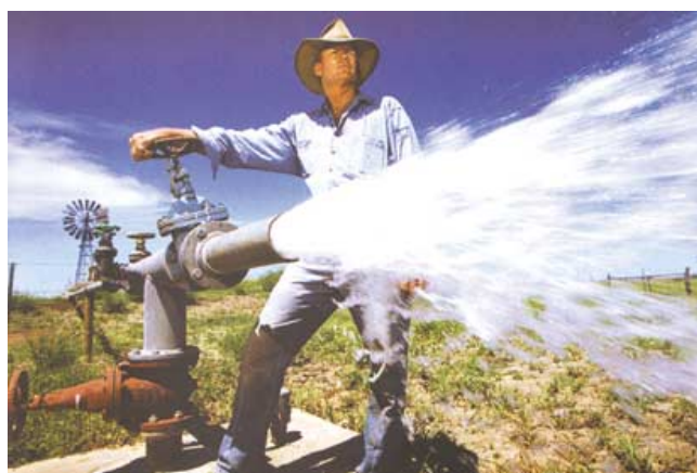
John Secombe, Chairman of the former Great Artesian Basin Consultative Council, demonstrating the volume of flow that is available at one bore at his grazing property near Longreach in Queensland. In this case the bore supplies hundreds of kilometres of distribution pipes. It is popularly accepted that the source of such flows is water seeping through porous sandstone at the base of the cased boreholes. That is evidently physically impossible. The author believes that the source must be high pressure steam in the jointed granite below the sediments, and that the steam flowing to the base of the bores has eroded the sediments to form a deep steam cavity down to the jointed granite which now supplies the borehole. (Newspix/David Sproule)
